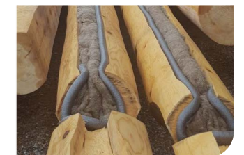
BLOCK PLANKING CONSTRUCTION
